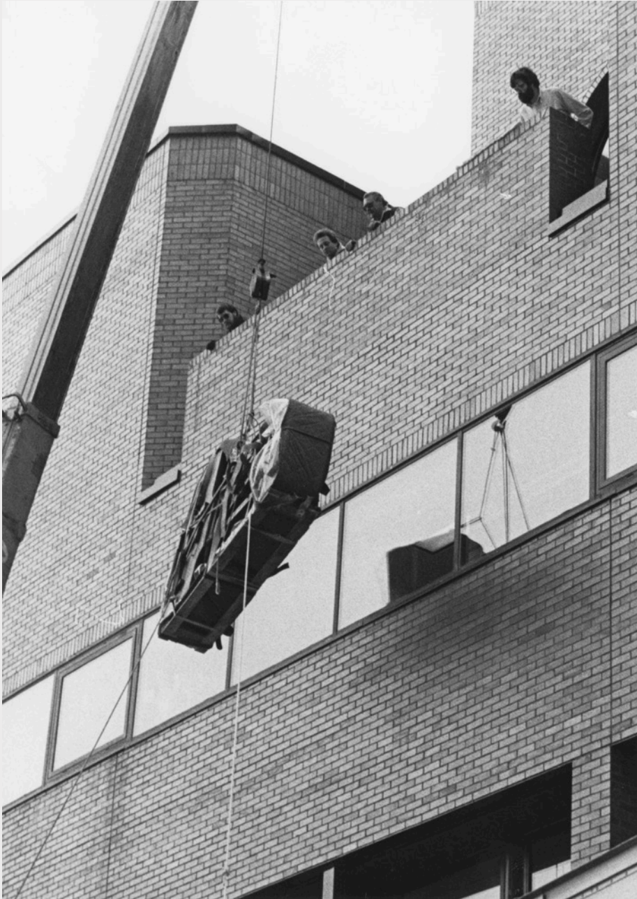
MPR staff watch as a piano is lifted by crane up to the Maud Moon Weyerhaeuser Recording Studio.
